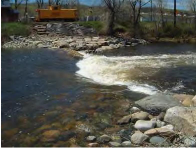
*Typical “U” Drop Structure in the Yampa River, Steamboat Springs, Colorado.*
